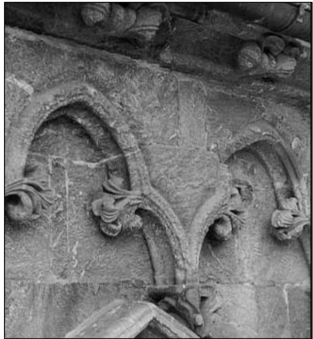
Fig. 22: Granular disintegration and delamination at a sheltered part of the south wall at Stavanger Cathedral. Former leaks may have brought large amounts of gypsum into the stonework.
