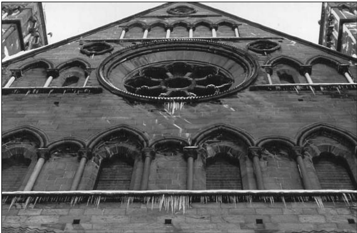
Fig. 12: Icicles forming from string courses made of Bjørnå stone, Nidaros Cathedral. The mouldings had recently to be removed due to dangerous cracks along foliation planes.
