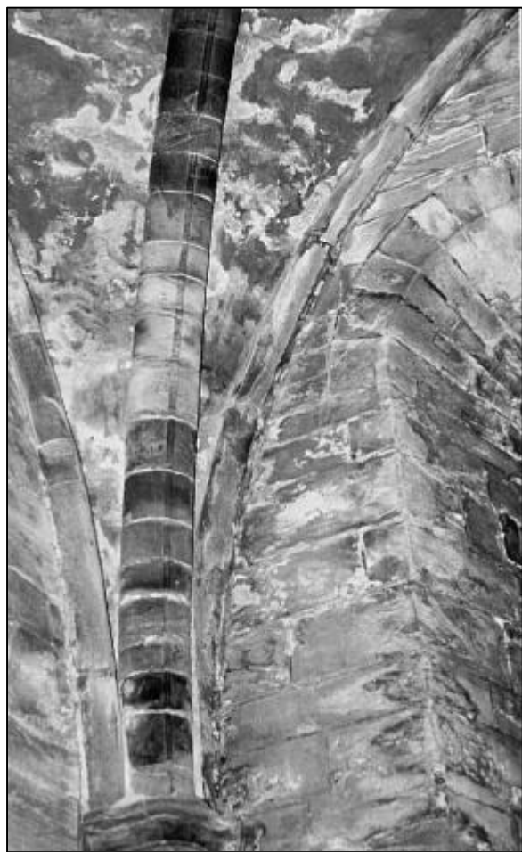
Fig. 20: West wall of the chapter house at Nidaros. The carbonate salt system consists mainly of trona and aphthitalite from cement mortars, but also some sodium sulphates can be found.
