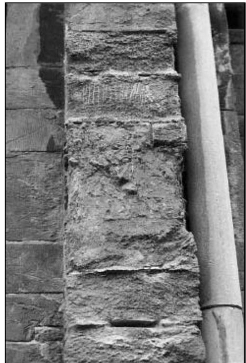
Fig. 15: Typical appearance of the worst damaged Grytdal stone.
