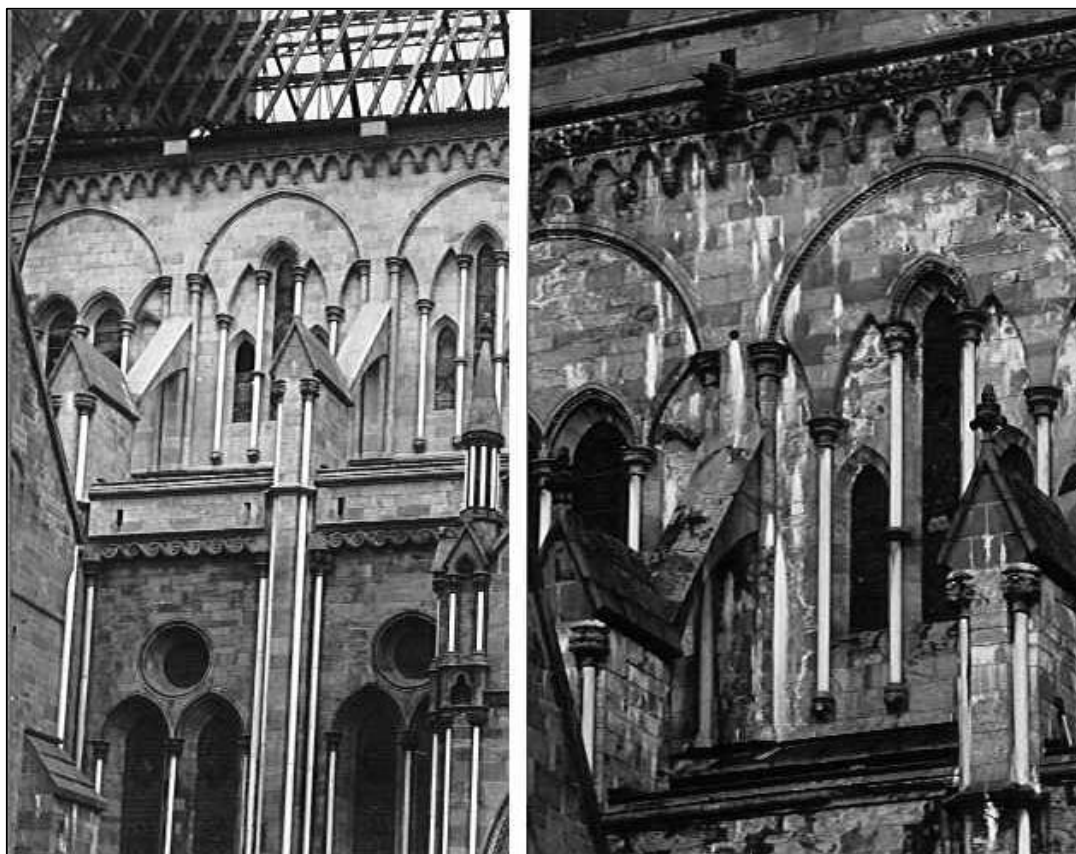
Fig. 23: The choir at Nidaros cathedral. Reconstructed in the 1880s (left), the choir today exhibits severe salt weathering (right). Salts present include calcite crusts, some sodium carbonates, but first of all gypsum, magnesium sulphates, sodium sulphates and a little chloride (secondary reaction system). The most important salt sources are Grytdal stone, brick in the inner walls and Portland cement mortars.
