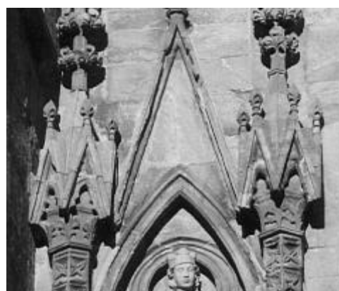
Fig. 14: Weathering at niches on the east front of Stavanger cathedral. Parts of mouldings are lost in the blind gable
