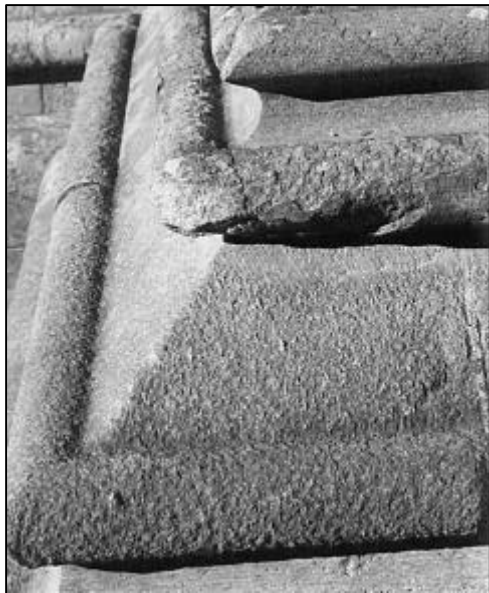
Fig. 9: Crumbling of exposed Bjørnå stone at Nidaros Cathedral
