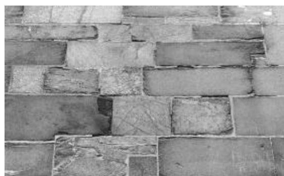
Fig. 5: Ashlars of Øye chlorite schist (dark) and Bakkaunet soapstone (light) side by side in the Octagon of Nidaros Cathedral. Note slight weathering along repointed cement joints.
