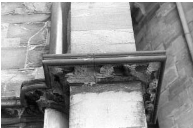
Fig. 13: Loss of carved detail underneath string course made of Øye stone, probably mainly due to the formation of black crusts.
