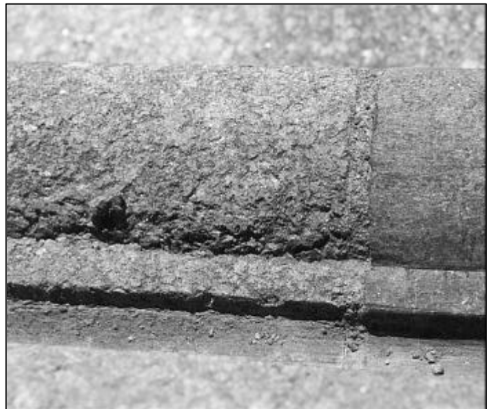
Fig. 10: Crumbling of exposed Bubakk stone at Nidaros Cathedral. The stone to the right is a serpentine
