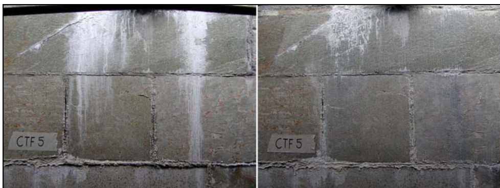
Before and after removal of calcite crusts (test field 5, south side of the choir).
