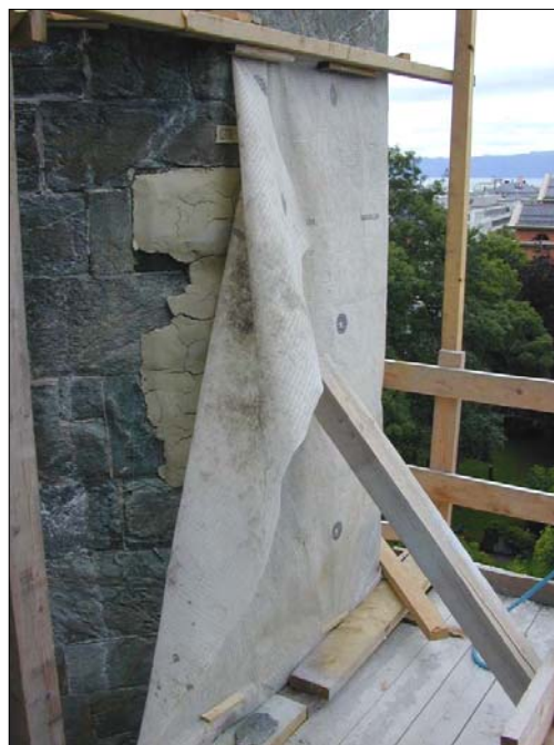
Dry two-layered desalination compress five days after application (test field 4, north turret of the choir)
