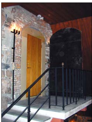
Figure 13: Temporary (reversible) door installed in the door-opening in the west wall of the Regalia room in February 2001
