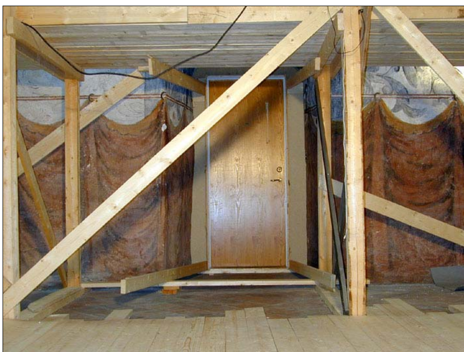
Figure 13: Temporary (reversible) door installed in the door-opening in the west wall of the Regalia room in February 2001
