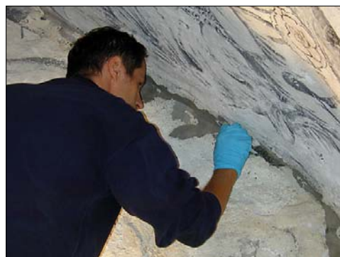
Figure 2: Closing cracks with lime mortar on the west wall in August 2001
