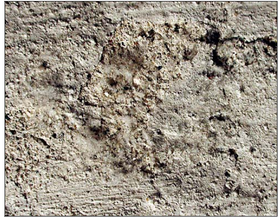
Figure 27: Long needles and whiskers of mainly halite and a little nitratine (sodium nitrate) forming cotton-like bundles. Width of photo: c. 8 cm. Photo no. RE02_003, sample no. RE130902_04. Microphoto no. RE02_010 (see fig. 22)
