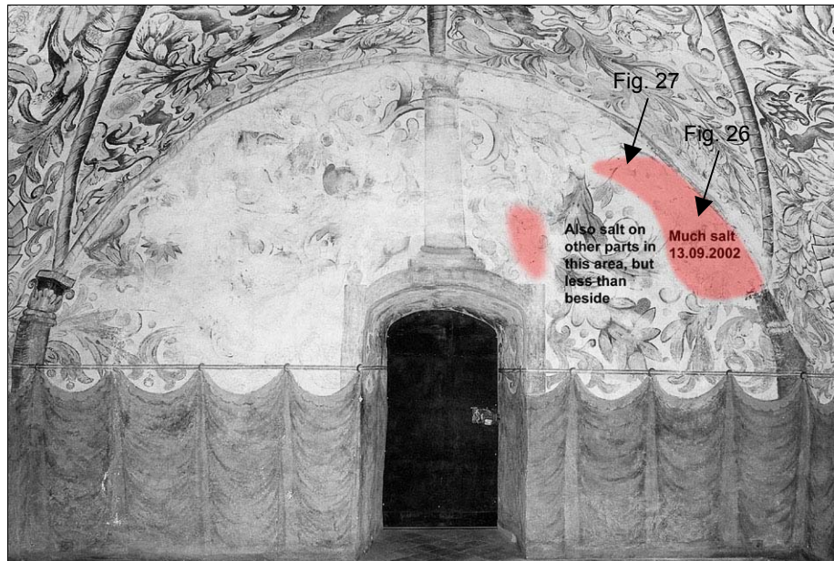
Figure 28: Areas with much salt in the middle of September 2002. Salts included mainly halite and nitratine.
