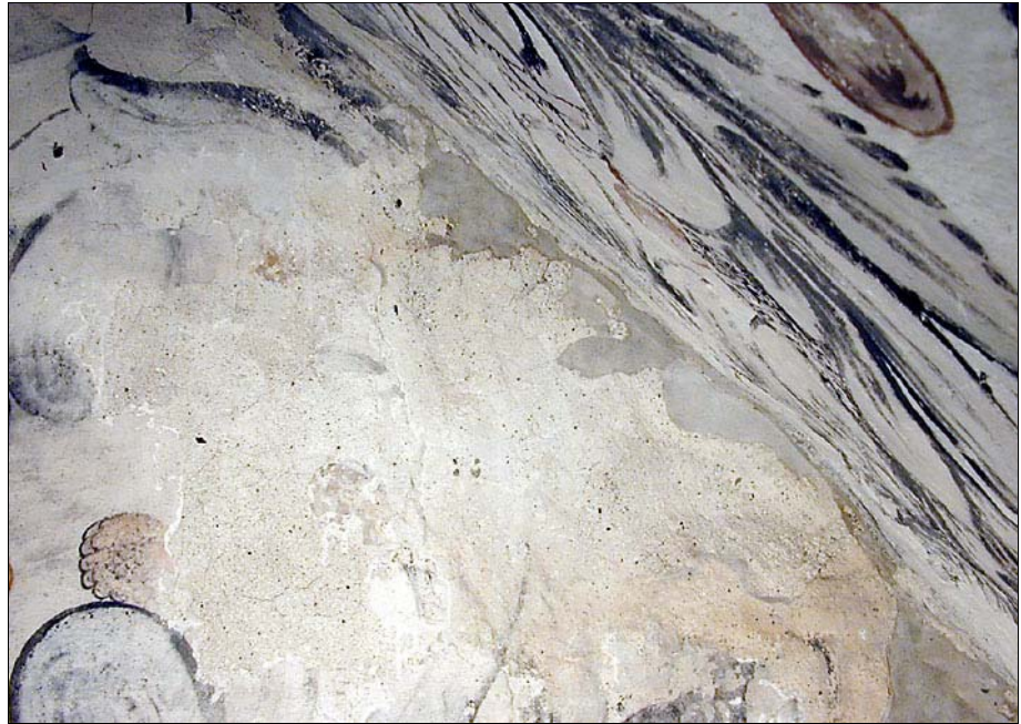
Figure 5: After application of lime mortar repair in the NW-corner
