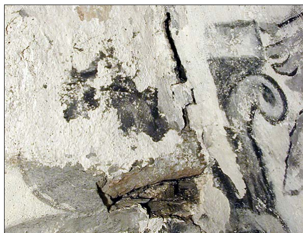
Figure 3: After removal of cement mortar from the 1966 restoration. NW-corner.
