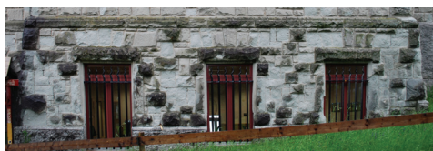
A heavily exposed part of the west façade in 2009. A few fragments (scales) had fallen down by 1975. The rest was knocked off mainly in 2005 and 2006 (light-coloured stones).
