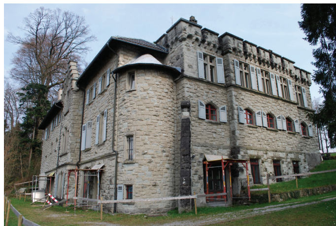
The "economy building" seen from the west with its two largest and most damaged walls in 2009. Lighter stones had their surfaces knocked off mainly in 2005 and 2006.
