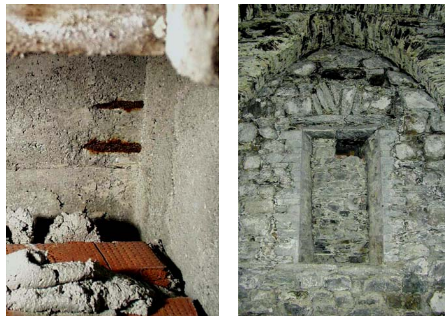
Two places where clues to the weathering in the Regalia room can be found. Left:: (Rusting) reinforced concrete inserted during the last restoration in the upper part of the opening at the rear of the northwest corner of the west wall. Right: The west wall of the vaulted room below the Regalia room. This room was used as gun powder store until 1826. Today there are massive amounts of alkaline salts of unknown origin on the walls
