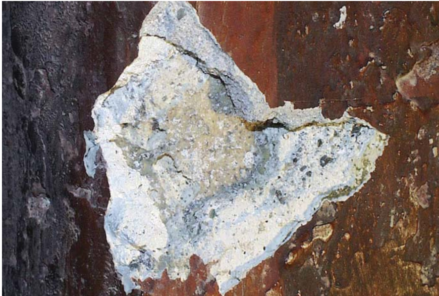
Mechanical damage at the south edge of the main door opening. On the "bottom" it is possible to observe a plaster from before 1616. The uppermost paint stratigraphy can be seen on the picture to the right.
