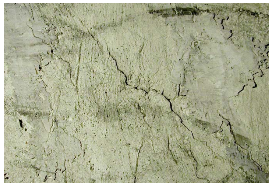
Crack pattern in the area above the door (type 3)
