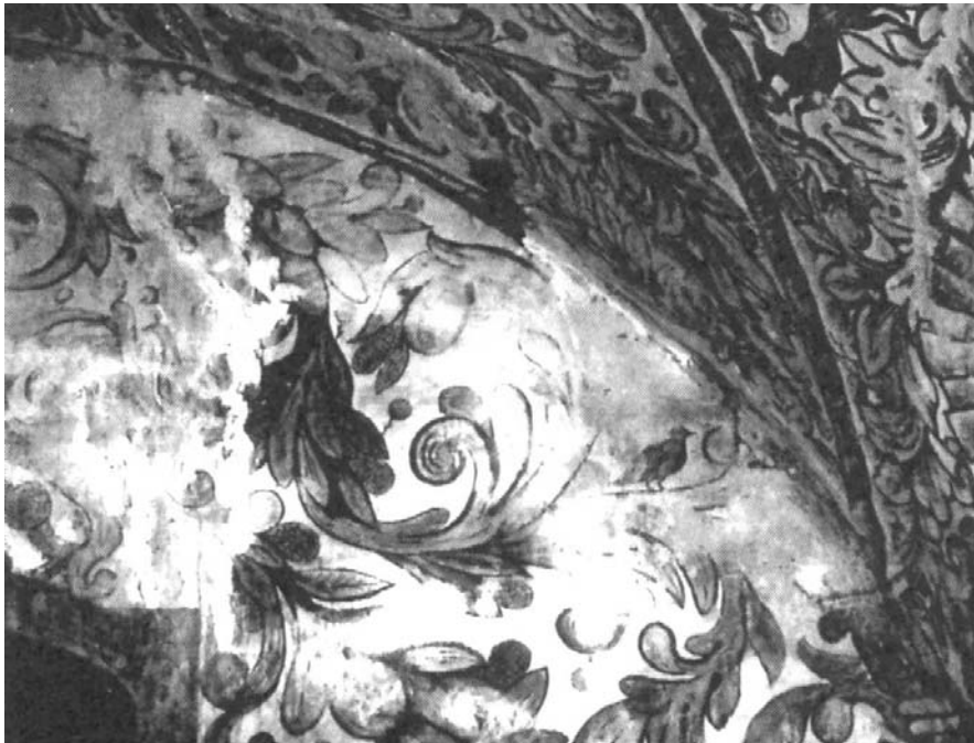
The west wall under restoration in 1966. Note all the white fields; many of these are gypsum repairs. (Photo: Archives of the Directorate for Cultural Heritage, Oslo)
