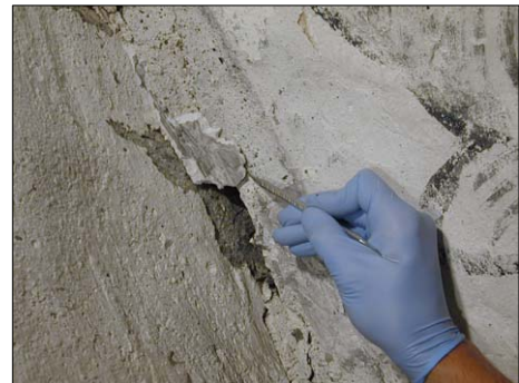
Removal of gypsum repair mortar from 1966 (in Q2)
