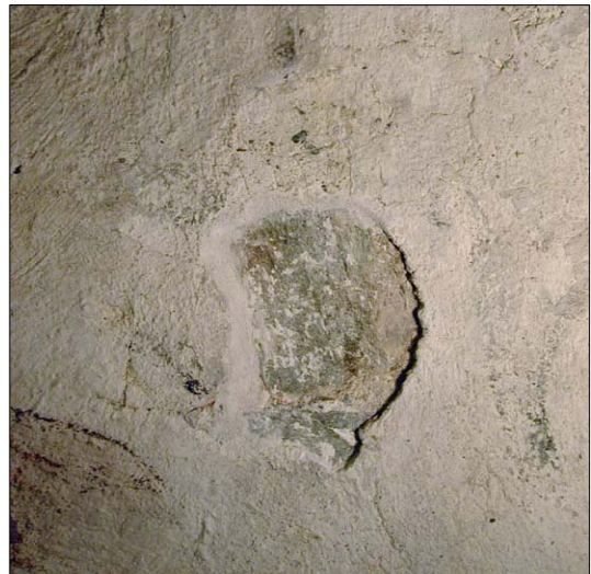
Upper right part of Q1. After removing a large gypsum repair hollow areas around were filled with lime mortar, which was also use to close the gaps around the "open" area. Salt crystal-lisation were observed after the work, but after being brushed away they did not return.
