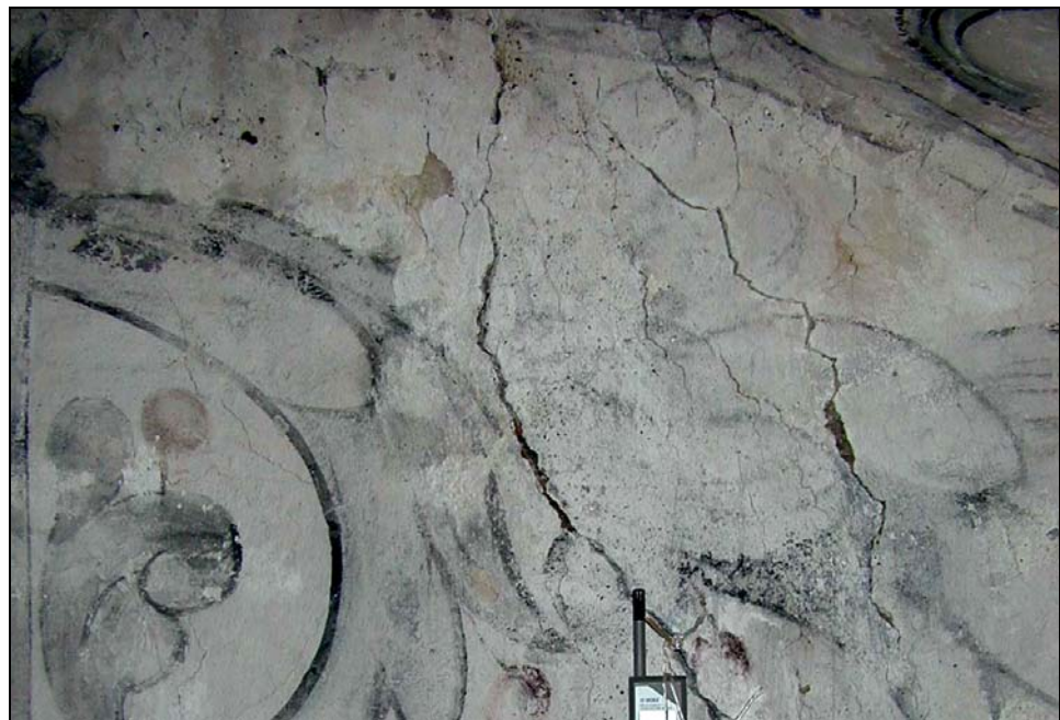
Cracks on the west wall (Q1) after removal of gypsum repairs from 1966. The cracks were closed with lime mortar in 2000
