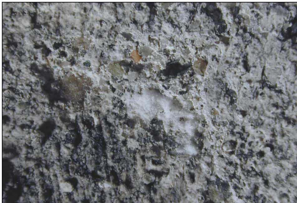
Powdery efflorescences and whiskers of epsomite in O.3. Width of field c. 5 cm
