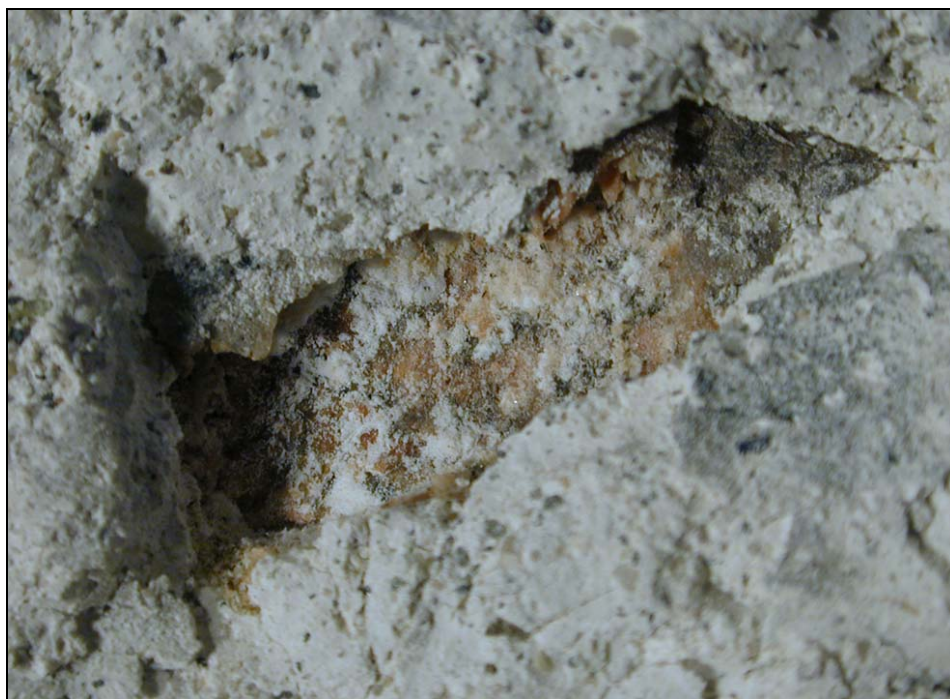
Observation spot O.2. Powdery efflorescences of thenardite. Width of field c. 5 cm.
