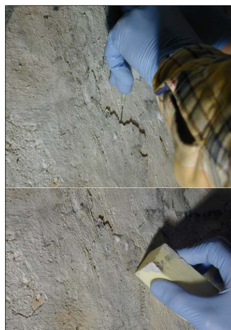
Injecting lime behind limewash
