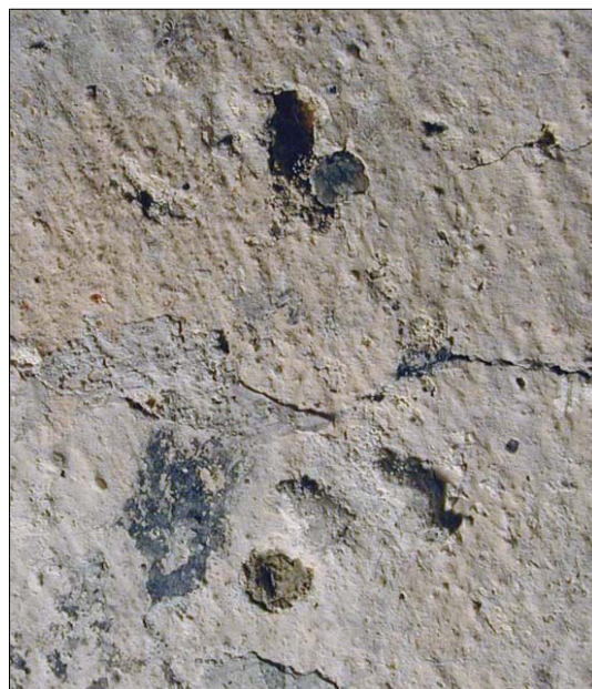
Holes for injection mortar (Q2)
