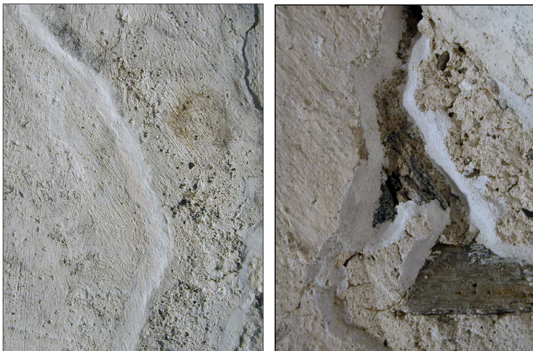
Closing of cracks and gaps with lime mortar in Q2. Right: Final closing of crack. Left: temporary closing of edges and corners (Q2).
