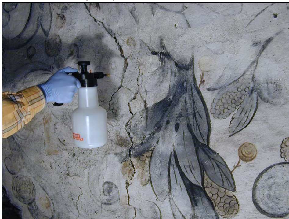
Spraying limewater on the wall in order to consolidate the surface (in Q2). Note also the extensive cracks, which appeared after the removal of gypsum repairs from 1966
