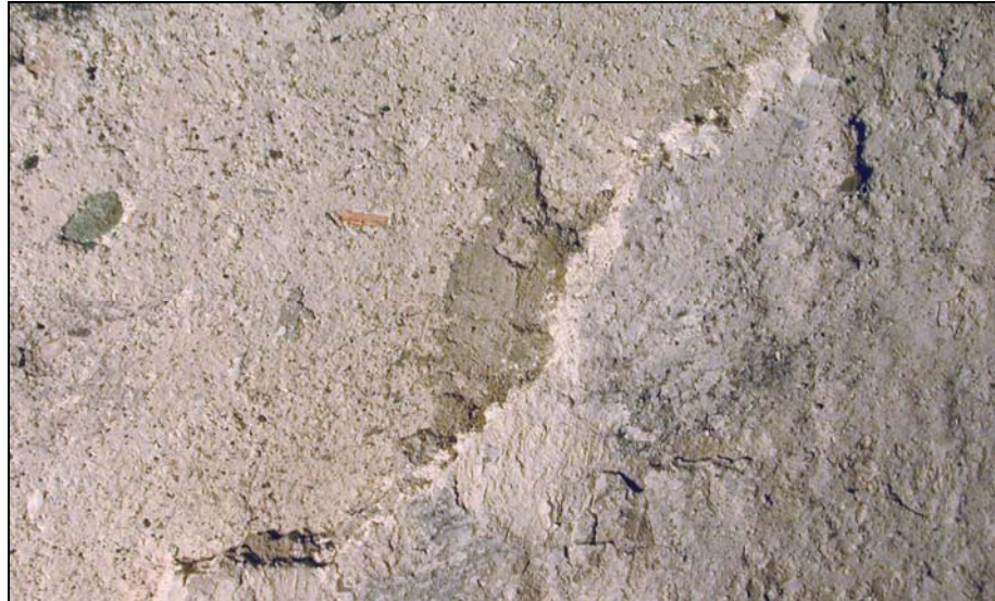
Gray injection mortar behind plaster in Q1
