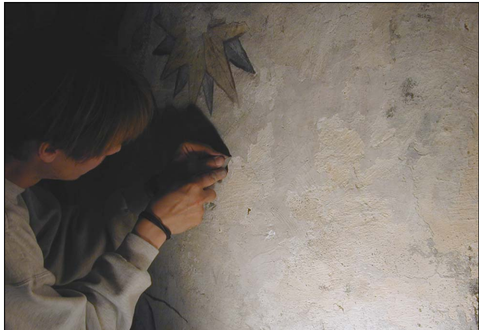
Removal of gypsum repairs "smeared" over the surface in Q1
