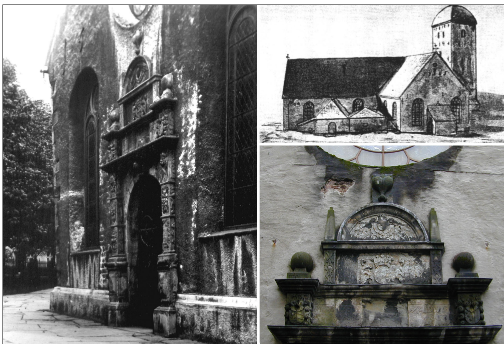
Figure 10: Church of the Holy Cross. Left: The north portal with much black crust by 1900. (Photo: Directorate for Cultural Heritage.). Top right: A porch in front of the portal in 1839. (Drawing by F. Bøe). Bottom right: The upper part of the portal in 1999, showing damages where crusts formerly prevailed.
