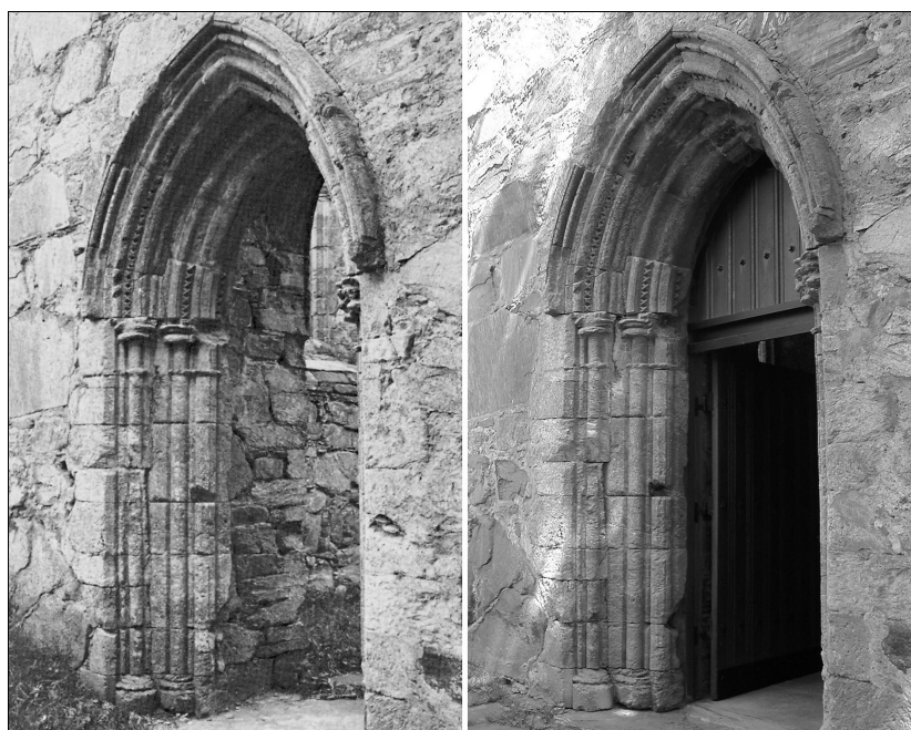
Figure 8: The west portal of Utstein monastery church before 1965 (Photo from [19]) and in 2001. Note many small damages and that the damages have hardly evolved.
