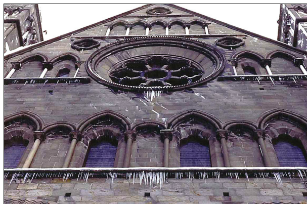
Figure 4: Icicles and snow at the S. transept of Nidaros cathedral. The stringcourses made from Bjørnå stone have lost their mouldings along the pronounced foliation in the stone. This stone has a lifetime of only 30-60 years when used at such places.
