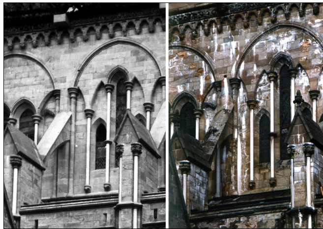
Figure 9: Left: The choir at Nidaros cathedral was reconstructed using much Portland cement and stone rich in sulphide (Grytdal) in the 1880s. (Photo: The Restoration Workshop of Nidaros Cathedral.) Right: 100 years of water leaks through the masonry have given massive calcite crusts and extreme salt weathering problems.
