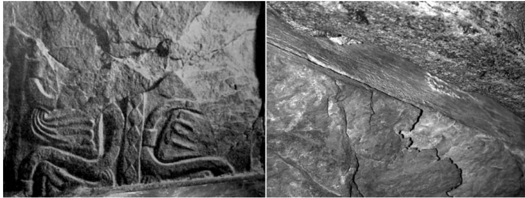
Figure 4: Left: The slab in the 1960s. Photo by the Restoration Workshop of Nidaros Cathedral. Right: An impression of the delamination of the slab.
