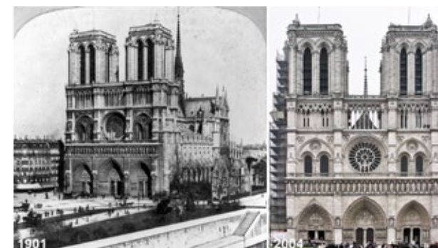
Figur 6. Notre Dame i Paris. Vestfasaden dekket av sorte skorper i 1901 (foto: Library of Congress, http://hdl.loc.gov/loc.pnp/cph.3b17261 ) og etter rengjøring i 2004 (foto: P.Storemyr). Notre Dame in Paris with the west façade covered by black crusts in 1901 and after cleaning in 2004.
