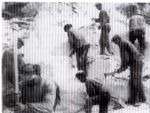
Figure 17 Quarrymen extracting soapstone blocks in the Gudbrandsdalen area in 1932. The work was undertaken almost as in the Middle Ages (after Voldheim, 1995).
