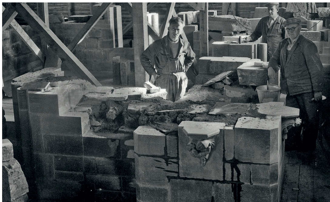
Fig. 6 Building the belfry of the southern west tower in the 1950s, using Portland cement mortars in both cores and joints. (Credit: Nidaros Cathedral Restoration Workshop)
