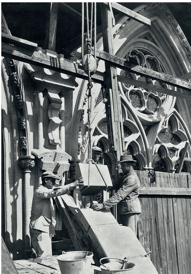
Fig. 5 Building the flying buttresses of the reconstructed nave in the 1920s, with buckets full of Portland cement. (Credit: Nidaros Cathedral Restoration Workshop)
