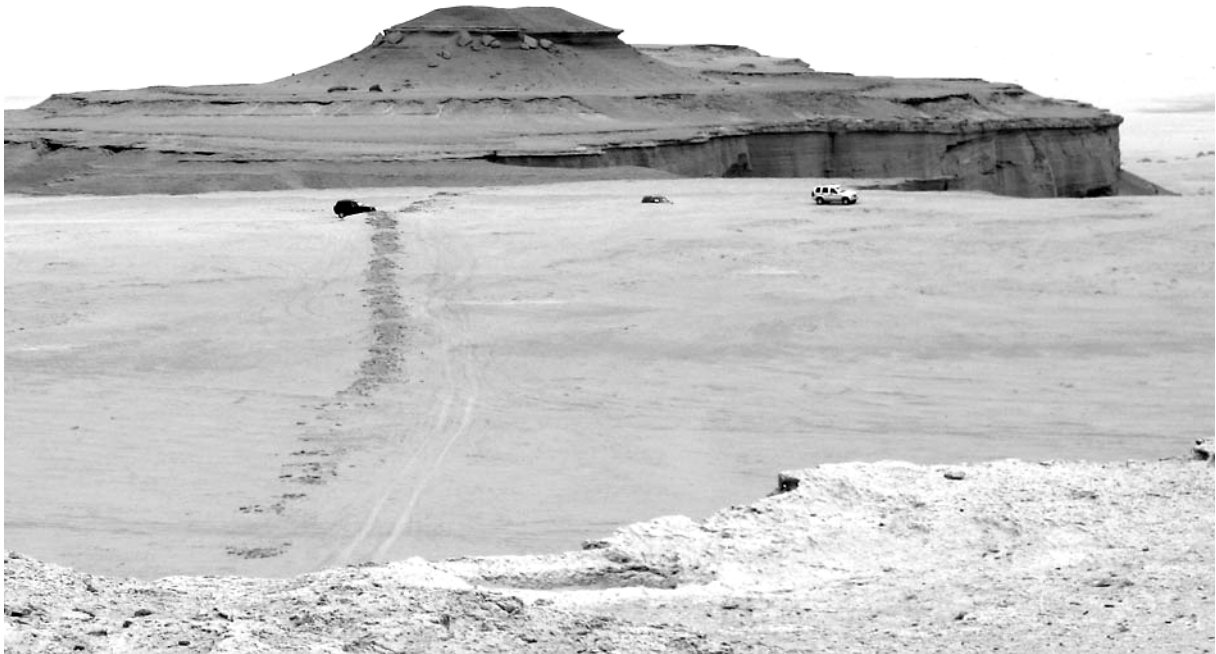
Figure 90: A portion of the Old Kingdom paved quarry road from Widan el-Faras to Qasr el-Sagha in the Northern Faiyum. This portion has been subject to wind deflation, causing that the road stands up from the surrounding sediments. This again leads to collapse of pavement slabs (photo: Per Storemyr 2006).
