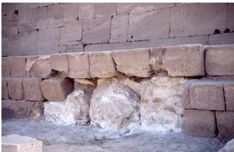
Figure 103: Weathering of Qurna limestone, probably from the Wadi el-Muluk quarry, in the temple complex at Karnak. Note that the limestone is much more susceptible to weathering than the surrounding Nubian sandstone. In this particular case the weathering is influenced both by naturally occurring salts (and clays) in the stone and salts provided by ground water (photo: Per Storemyr 2001)
