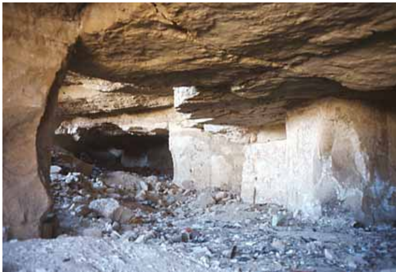
Figure 102: Underground gallery in the Wadi el-Muluk quarry. Salt weathering predominantly takes place along the lower reaches of the walls (photo: Per Storemyr 2001)
