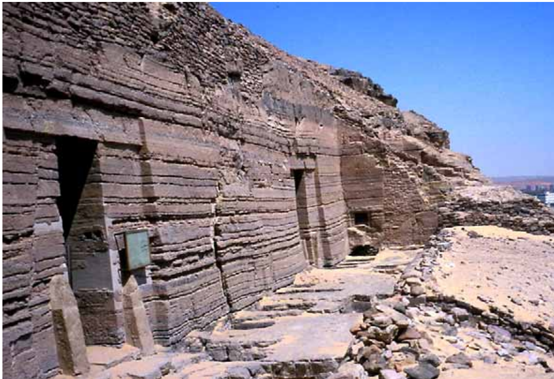
Figure 104: Differential weathering in the sandstone faces of the Tombs of the Nobles on the West Bank of the Nile at Aswan (photo: Per Storemyr 2001)
