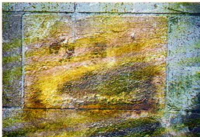
Fig. 2. Colour contrast between heavily deteriorated (brown/red/yellow) and less deteriorated (grey) soapstone on the outside wall of the Nidaros Cathedral. The intact (not deteriorated) soapstone is black in colour.
