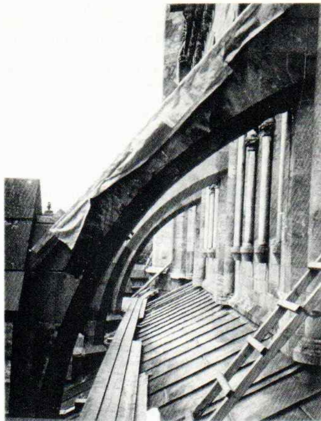
Fig. 15. Flying buttress from the Nidaros Cathedral showing a variety of deterioration states.
