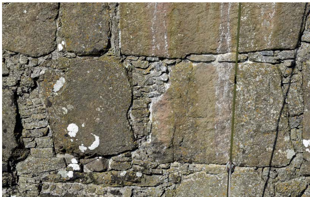
Fig. 8. The rubble masonry at the east end of the cathedral, with widespread use of pinning stone in vertical joints. Photo Per Storemyr 2017.
