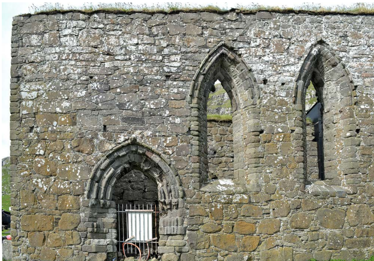
Fig. 4. The rubble masonry of Múrun, showing the portal and windows in the south-western part of the nave. Note large, polygonal stones lower down and more slab-like stone at higher elevations. Photo Per Storemyr 2017.
