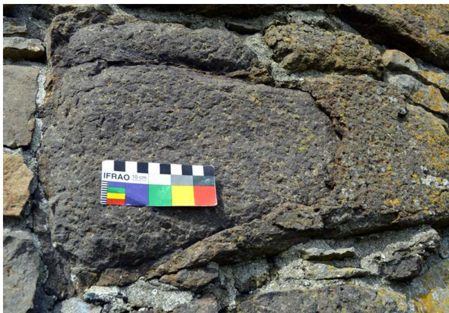
Fig. 10. A basalt block with pronounced spheroidal weathering at the south facade of Múririn. Photo Per Storemyr 2017.
