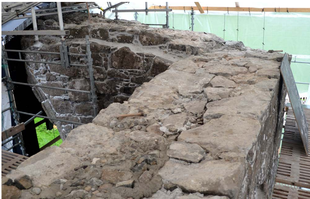
Fig. 7. The south-eastern wall-head under restoration in 2017. There are slab-like blocks and a very narrow core with little mortar. Photo Per Storemyr 2017.
