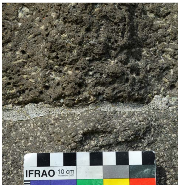
Fig. 11. Typical decorative stones at Múririn: Greyish and brownish/purplish soft basalt, both porphyritic. West portal in the south façade. Photo Per Storemyr 2017.
