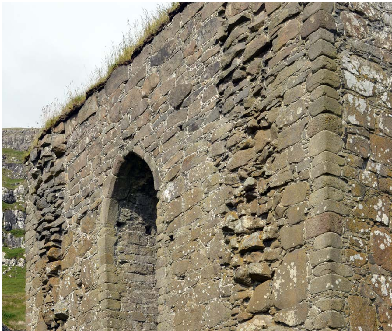
Fig. 6. The western facade with the remains of masonry belonging to the vanished tower. The quoins have been worked into rectangular forms. Photo Per Storemyr 2017.
