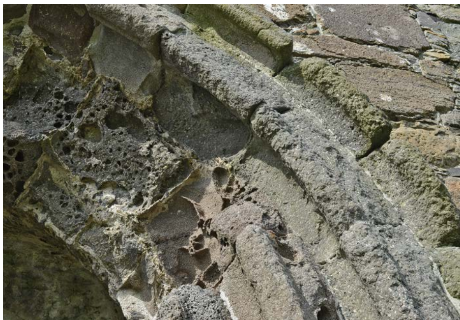
Fig. 12. Extreme cavernous weathering (tafoni) of soft decorative stone. West portal in the south facade. Photo Per Storemyr 2017.
