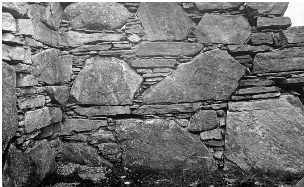
Fig. 9. Rubble masonry with widespread use of pinning stone at Selja Monastery, western Norway. Photo The Norwegian Directorate for Cultural Heritage.
