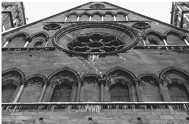
Fig. 4. Icicles and snow at the S. transept of Nidaros cathedral. The stringcourses made from Bjørnå stone have lost their moldings along the pronounced foliation in the stone. This stone has a lifetime of only 30–60 years when used at such places.
