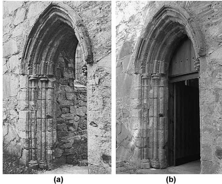
Fig. 8. The west portal of the Utstein monastery church (a) before 1965 (photograph from Ref. [19]) and (b) in 2001. Note many small damaged areas and that these damaged areas have hardly evolved.
